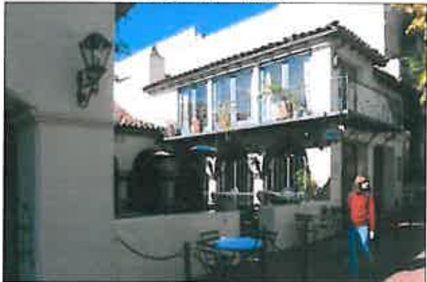
Commercial forecourt provide outdoor dining area along a vibrant commercial street. The ROW is defined by a low wall as required by the code.
