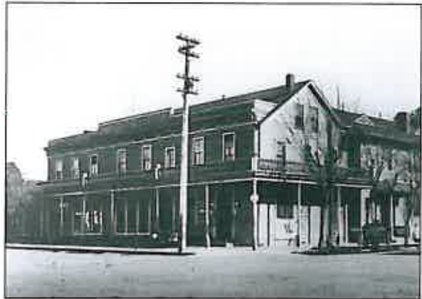
Historic Livermore commercial block type with gabled roof form and gallery.
