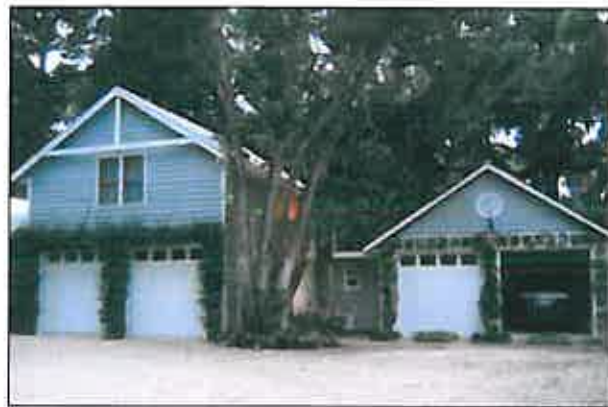
One-and-a-half-story carriage house next to a two-car garage.
