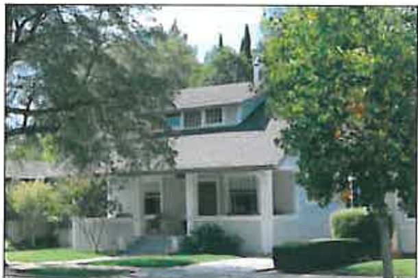
Full-length integral porch integrated into the overall massing.
