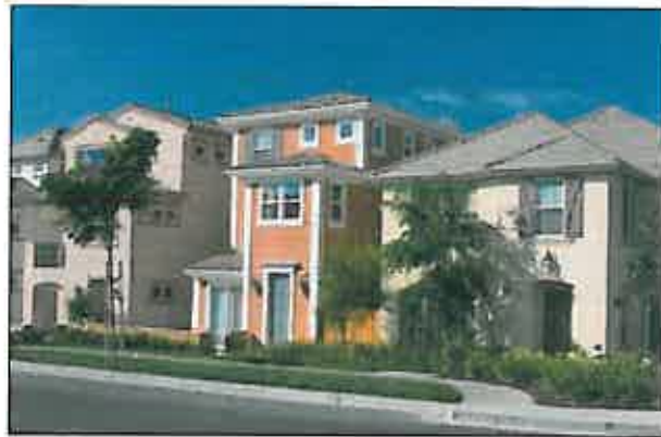
Newly constructed small lot single-family home in Livermore.
